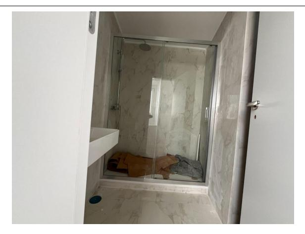
Building on the progress made in August, the construction team continued installing sanitary fixtures in the apartment bathrooms throughout September and October. This included the installation of shower trays and glass doors, washbasins, and faucets. The team ensured all fixtures were properly aligned and securely installed, adhering to both functionality and design standards to create modern, high-quality bathroom spaces.
