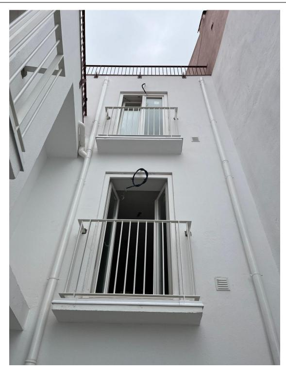
The balcony guardrails were produced in September and delivered to the site. The builders then proceeded to install them on each apartment balcony, ensuring both safety and aesthetic appeal. These guardrails not only provide essential protection but also enhance the overall design of the balconies.
