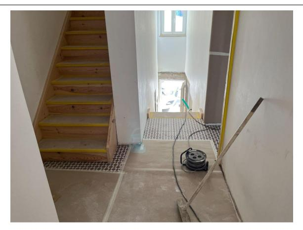
The installation of the staircase was completed, both in the apartments for interior use and in the common areas. Following this, the builders began tiling the common area floors with ceramic tiles, carefully applying a classic pattern to enhance the aesthetic appeal and durability of the spaces.
