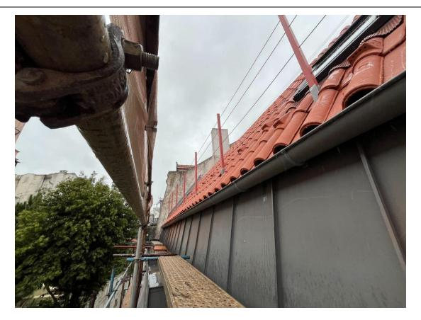
The zinc cladding work progressed steadily and was successfully completed by September 17th. This durable cladding was meticulously applied to provide a weather-resistant exterior finish while enhancing the building's architectural appeal with its decorative qualities.
