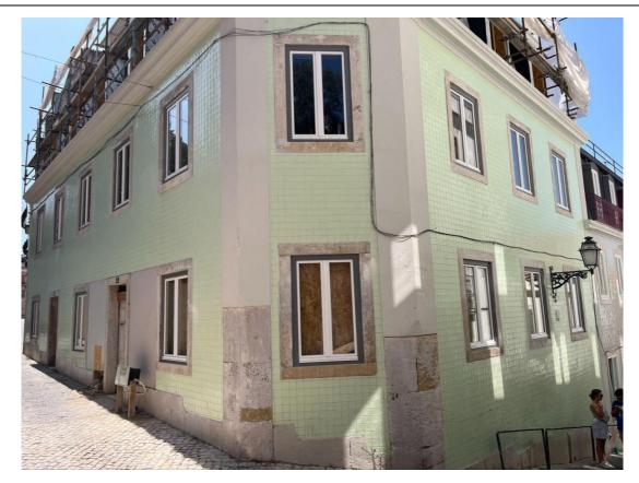
As noted in the previous report, the construction team began installing windows in the apartments on the ground and 3rd floors. In August, they completed the installation of windows on the ground, 3rd, and 1st floors carefully.
