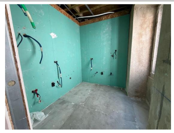
As mentioned in the July report, the construction team was installing insulation within the interior walls on the ground and 3rd floors, as well as beginning to place gypsum boards on the walls of the 1st floor.
