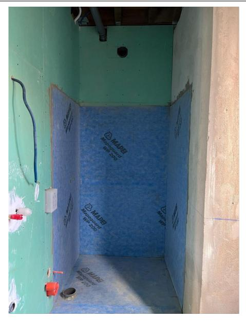
Building on the work completed last month, the construction team continued their efforts in the kitchen and bathroom areas in August. After finishing the installation of backplates on the floors, they applied a primer layer to the backplates to enhance surface preparation. Following this, they began applying a waterproof layer to both the floors and walls.
