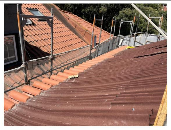
As mentioned in the previous report, the construction team was focused on the roof. They successfully completed the installation of panels on the roof's steel structure and proceeded to place the sub-tiling materials on these panels in preparation for the final tiling in July and August. Following this, they began tiling on the eaves in August.
