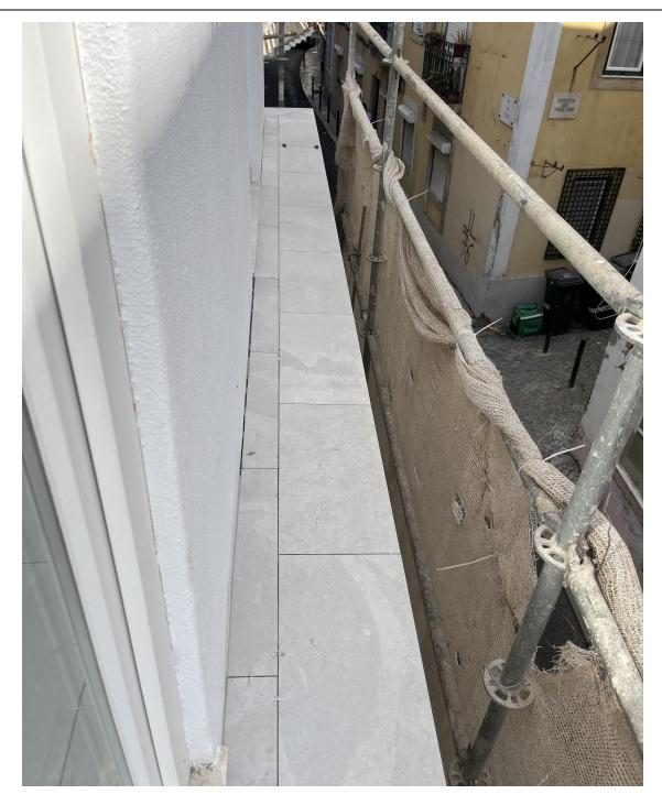
Meanwhile, the construction team was leveling the balcony floors in preparation for tiling. In July, after the tiles were delivered, they began the tiling process on the balconies.
