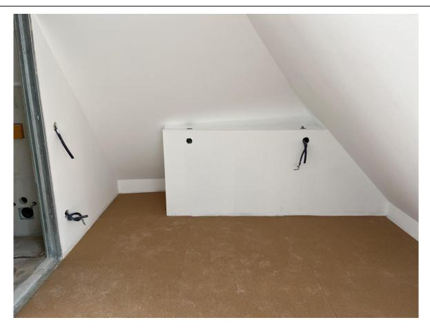
Following the work agenda, in July, the installation of flooring insulation commenced in July, starting from the 3rd floor and progressing downward to the ground floor. The insulation material used is cork, chosen for its soundproofing and thermal insulation properties. By the end of the month, the team had meticulously completed the installation on both the 2nd and 3rd floors.
