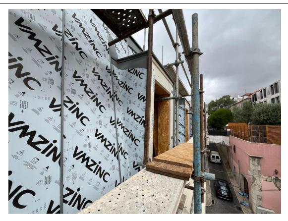
Following the work in June, the builders continually progressed with zinc cladding and roof tiling on the street-facing side, as well as placing insulation on the facade.
