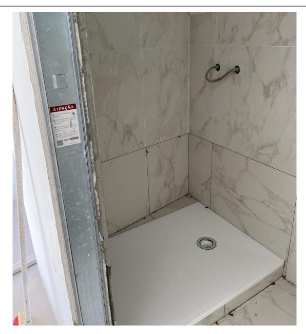
As mentioned in the previous report, the builders finished applying waterproofing to the bathroom areas of the apartments and started tiling the floors and walls of the bathrooms. In June, they were tiling the bathrooms and installing shower trays for all apartments in the Passadiço project.
