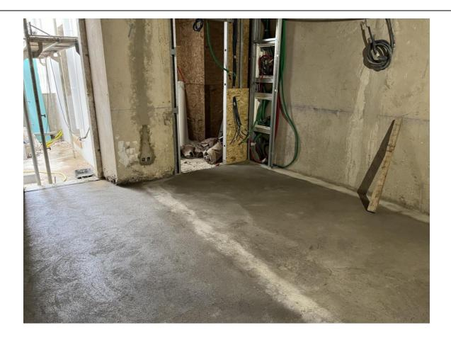
In June, the builders started to do screeding on the ground floor, placing a top layer of material laid over the concrete subfloor, to smooth the floor slab and assist in flattening.
