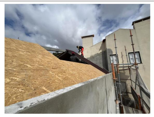
In June, the construction team concentrated on advancing the roof work. After assembling the roof steel structure, they proceeded with installing panels on it. By the end of the month, they started placing the sub-tiles on the panels in preparation for the final tiling.
