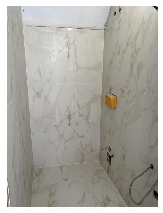
As mentioned in the previous report, the builders began applying waterproofing to the bathroom areas of the apartments above the ground floor, preparing them for the upcoming tiling phase. This month, they started tiling the floors and walls of the bathrooms.
