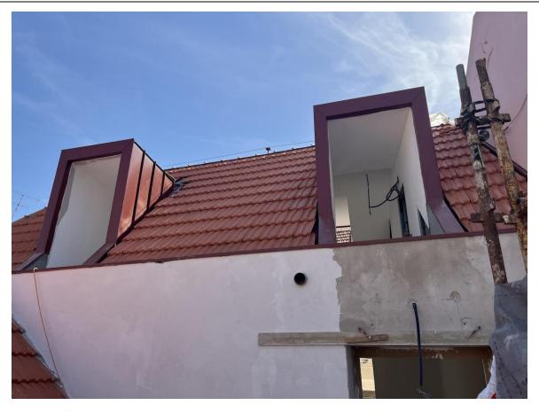
In May, the builders finished the roof tiling and also completed placing zinc cladding to cover the edge part of the roof.
