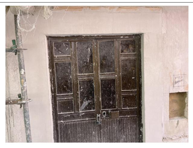
In compliance with the regulations governing rehabilitation projects in Portugal, it is mandatory to preserve the facade structure of the building. In May, the builders focused on repairing the existing stone window frames as part of the project. This essential work was undertaken to ensure the frames were properly prepared for the installation of new window scheduled for June.
