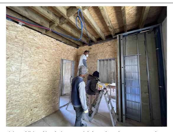
After receiving additional insulation materials by orders, the constructors began placing insulation not only on the facade but also within the interior walls of the apartments on the 1st floor. They then completed the wall structure by installing the second panels.
