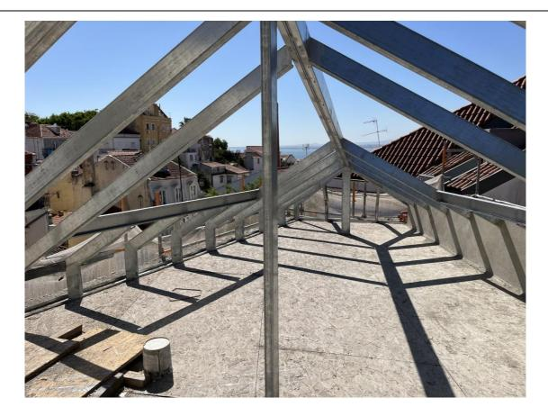
As mentioned in the previous report, the builders began assembling the steel structure for the roof in April. This month, they concentrated on completing this assembly, successfully installing the steel structure frame on the roof and constructing the surrounding walls along the roof edge.
