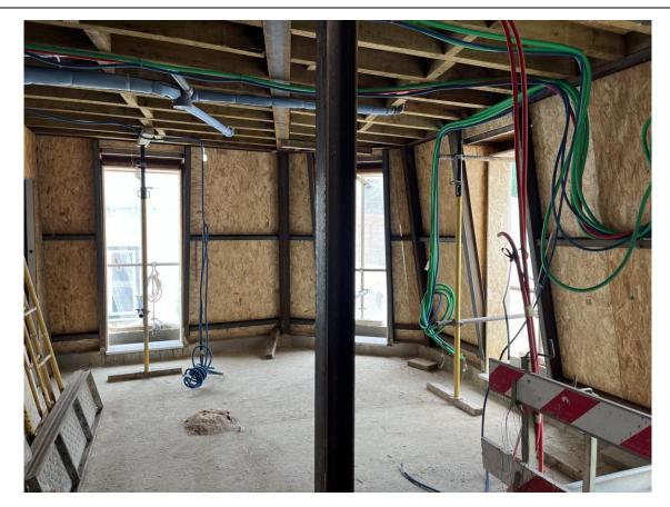
Following the work completed in April, the builders finished installing panels for the 2ndfloor facade. Subsequently, they began placing insulation materials on the facade to protect against heat. Meanwhile, the builders also worked on forming the rainwater drain channel for storm drainage on the 2nd-floor and applied waterproofing to it.
