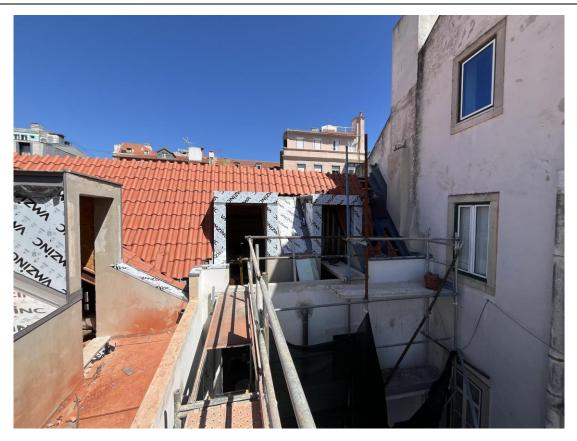
As mentioned in the previous report, the builders commenced work on the zinc roofing and cladding, alongside roof tiling, in March. In April, they continued with the roof tiling, completing the zinc covering and roof tiling on the side that facing the garden.
