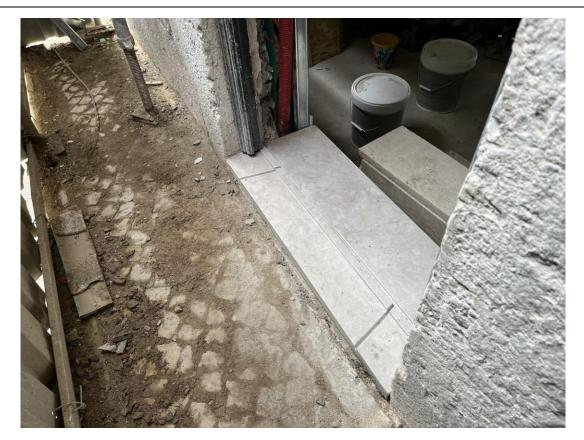
Meanwhile, the construction team initiated work on the zinc roofing and cladding in accordance with the design specificaations for finishing. Additionally, they began placing stone sills on all the windows and doors of the various sections in March. It's worth noting that the windows were being produced and pre-assembled in the factory workshop.
