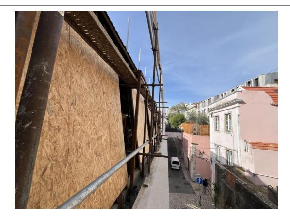
Following the work undergoing in the preceding report, the construction team diligently completed the assembly of the steel structure for the mansard windows by March. Subsequently, the builders proceeded to install panels for the dormer windows and the facade. Furthermore, they initiated the laying of stone sills for the window framework to enhance both aesthetics and functionality.
