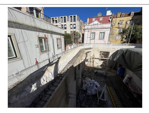
As mentioned in the last report, the builders demolished the upper walls a bit more to prepare for the capping beam made of steel and concrete, which tiles all the piling together to create the foundation for the next step. In September, they continued installing the columns and bricks on the beam to rebuild the external walls of the building facing the garden. Meanwhile, they started to prepare to build capping beams on the front façade walls.
